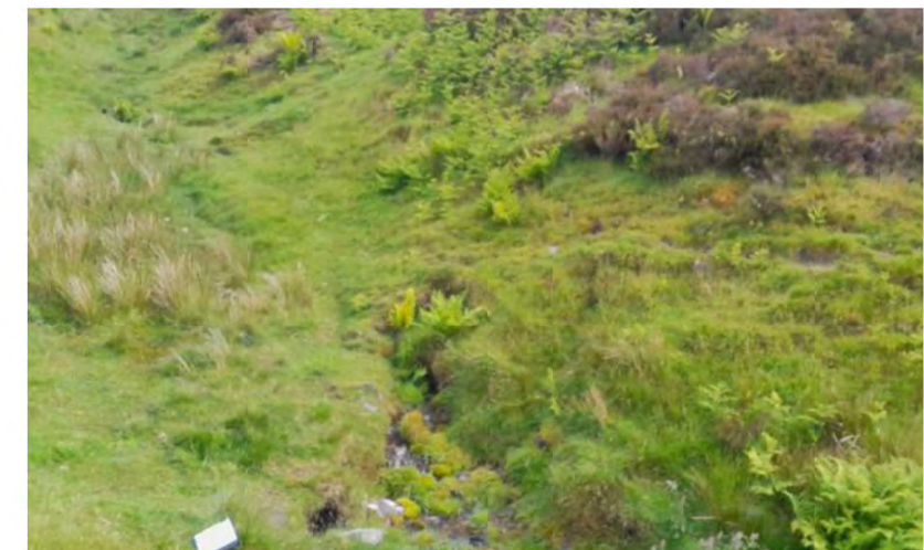
Photo 6: Water issuing from collapsed drainage adit on Bulmer Vein – Overcleuch Mine
