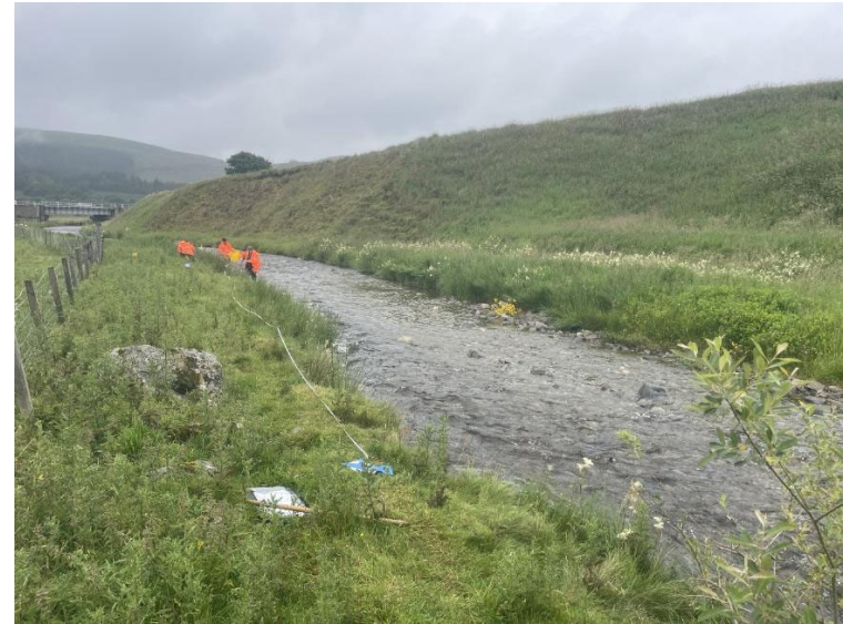
Plate 12: Site CEL010F, Elvan Water, Elvanfoot
